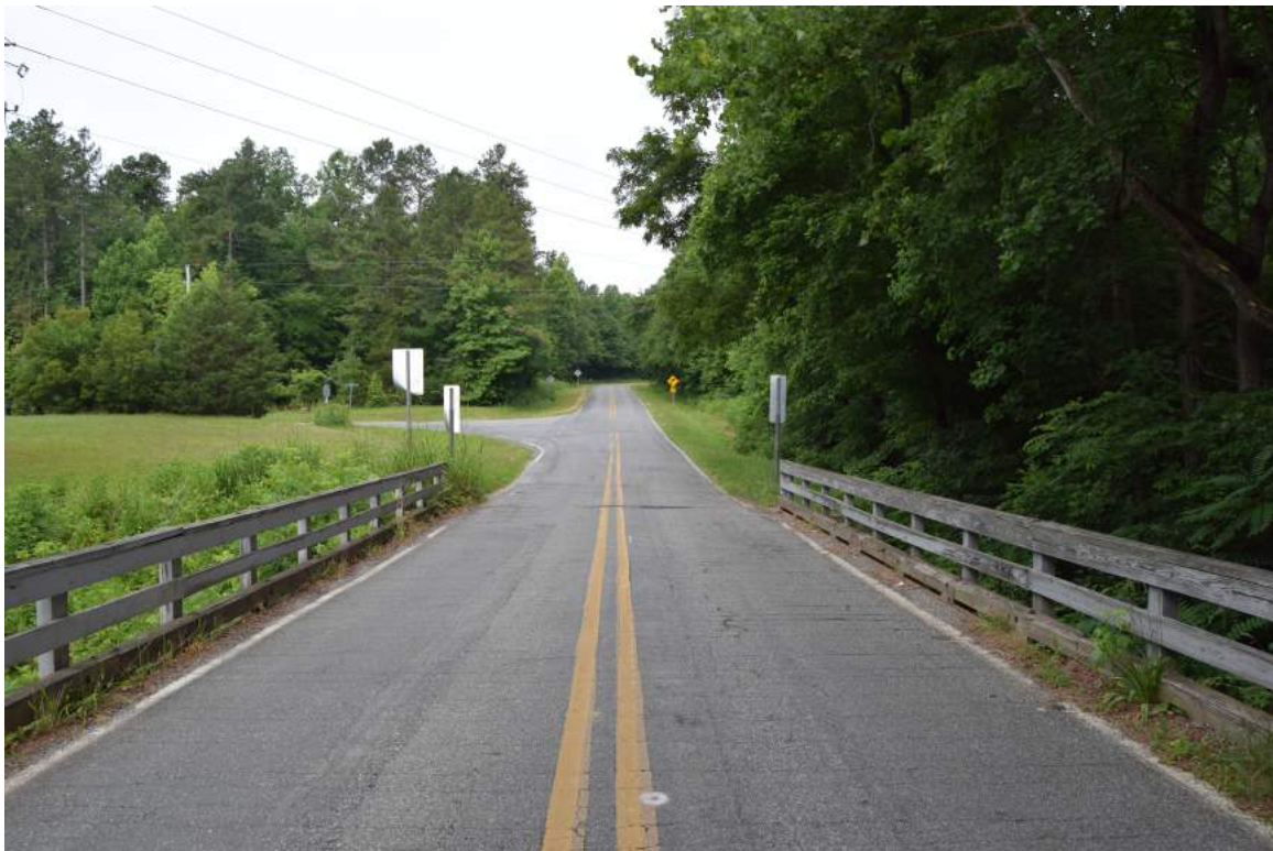
View along Hall's Mill Road, looking west from Bridge 11
