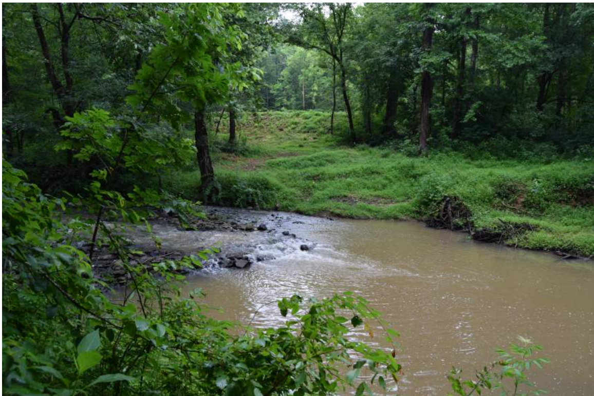
Hall's Mill Site (OR0906) Dam Ruin, view east from west bank
