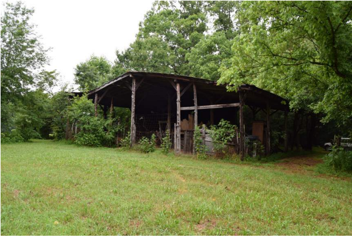
Pole Barn (OR2914), view to northwest
