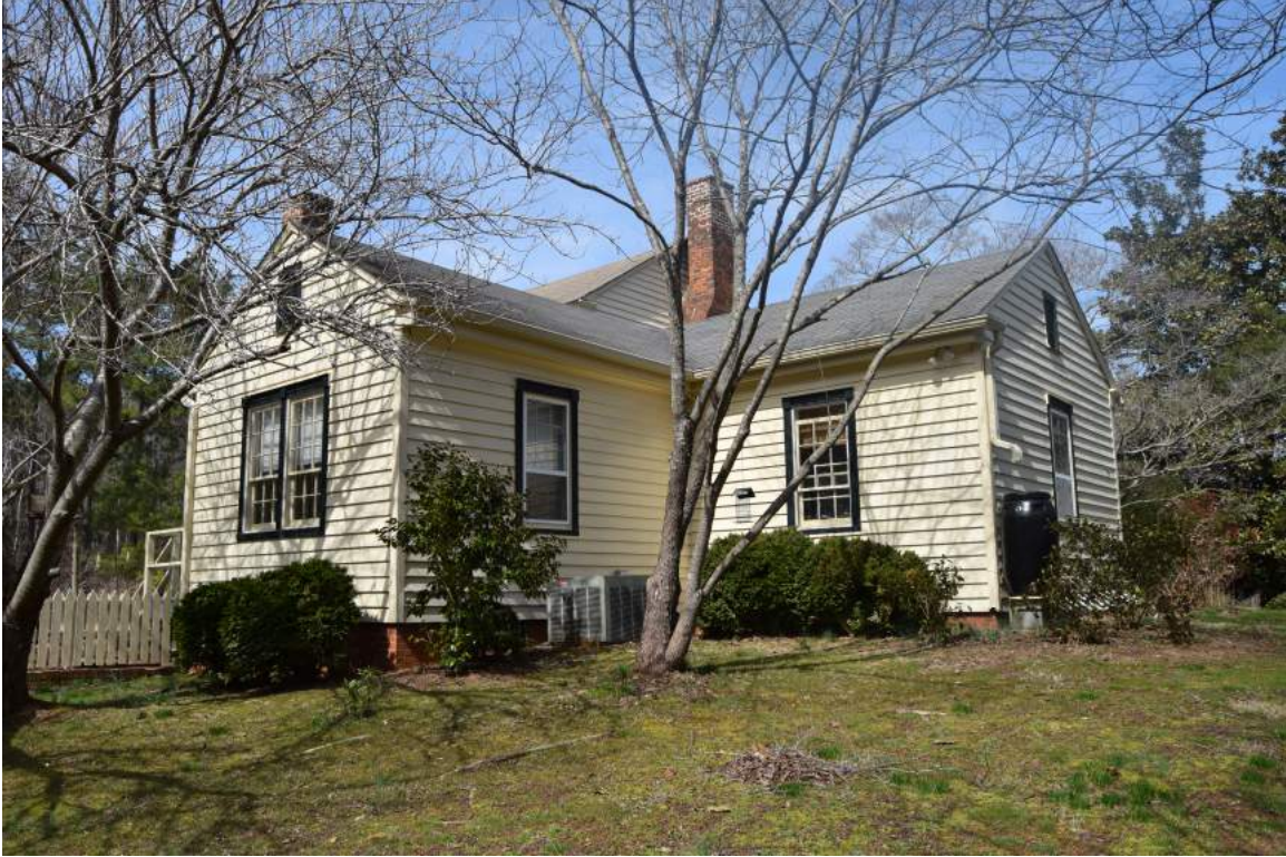
David Faucette House (OR1276), showing 1970s addition, view from rear yard to northwest.
