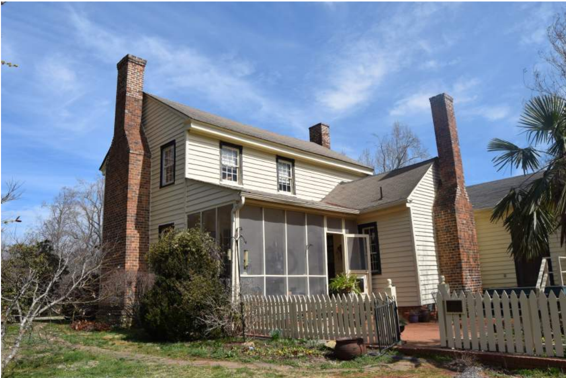
David Faucette House (OR1276), rear elevation, view from rear yard to northeast.
