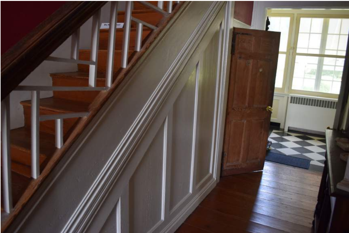
Moorefields (00010) interior, photographed September 2015 by the authors
