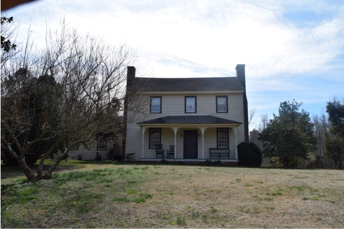
David Faucette House (OR1276), façade, view from front yard to south.
