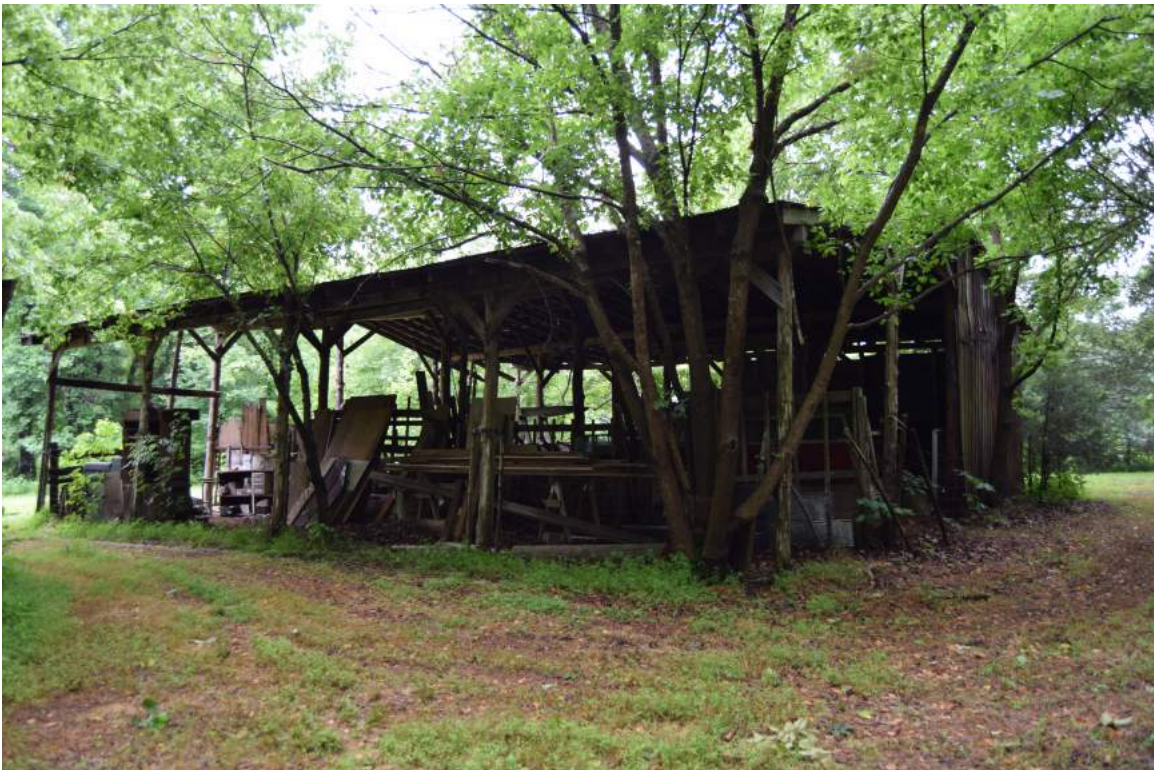
Pole Barn (OR2914), view to southwest
