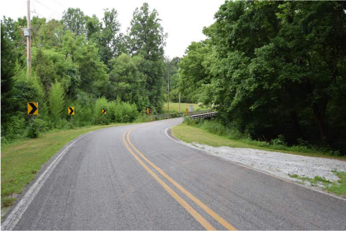
View along Hall's Mill Road, looking west toward Bridge 11
