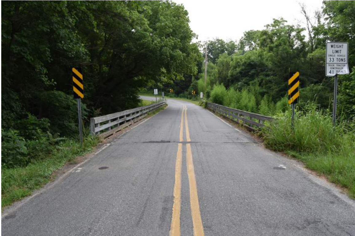
View along Hall's Mill Road, looking east toward Bridge 11
