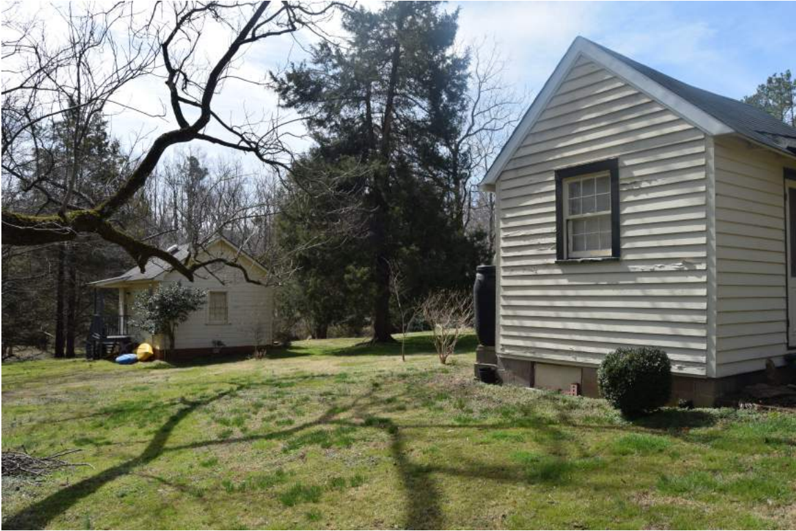
David Faucette House (OR1276), two moved outbuildings in the rear yard, view southeast.
